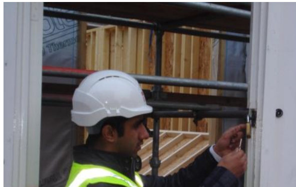
Officer Securing Site Compound
